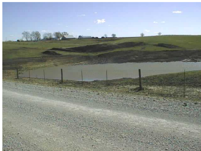
Installed road structure in the Rathbun Lake watershed, Wayne County.
